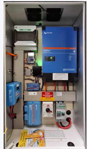
Victron inverter, MPPT, BMS and wiring
